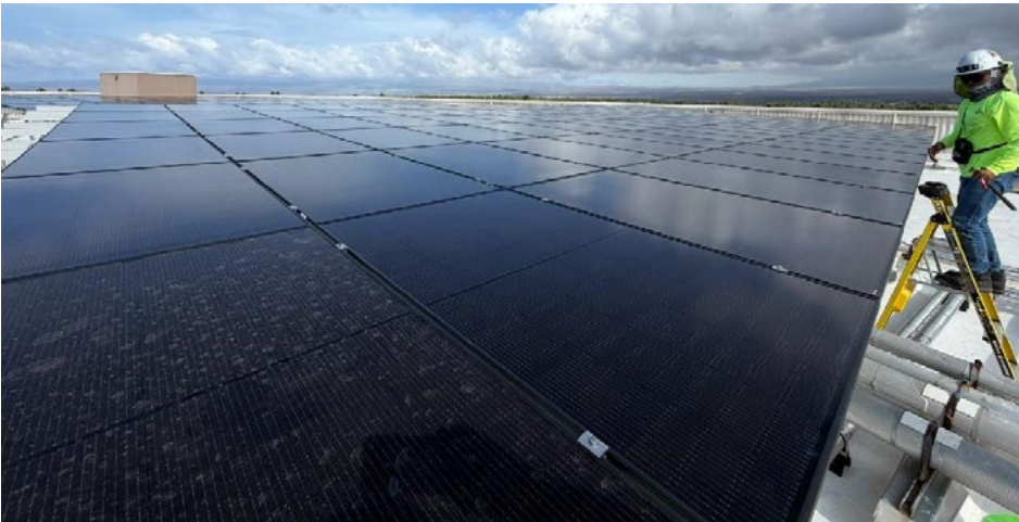
Solar PV panels installation
