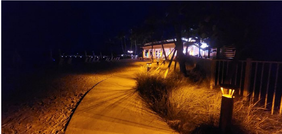
Solar bollard installation at Casa Marina
