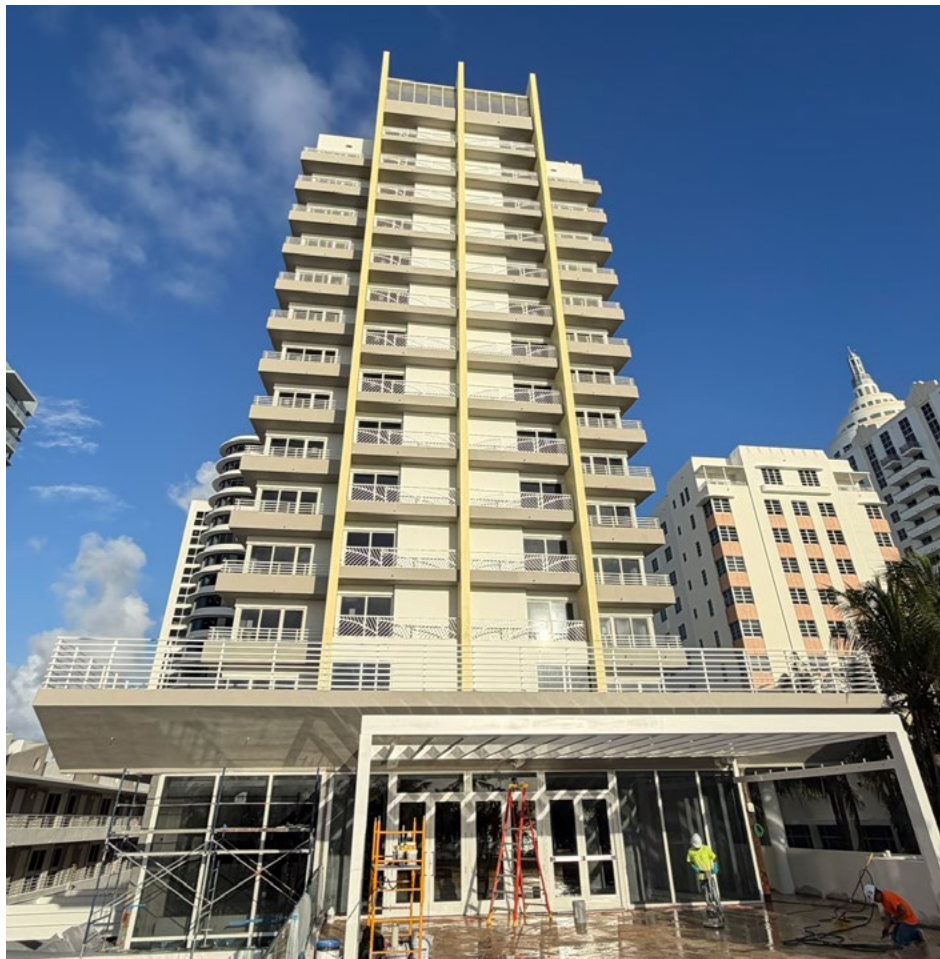
Exterior construction at Royal Palm
