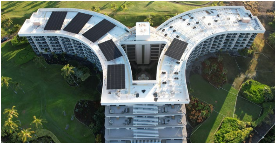
Solar PV panels installation progress on Palace Tower
